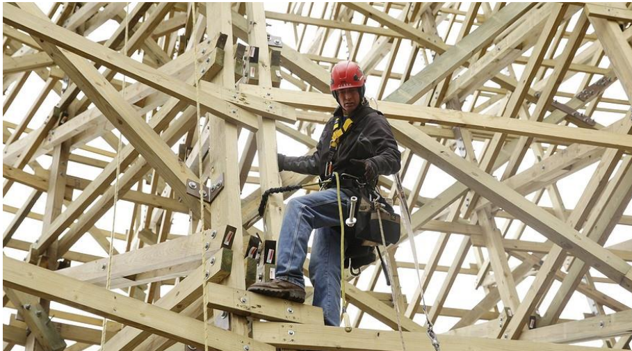
Curtis Clark works high up on the new Goliath roller coaster under construction at Six Flags Great America in Gurnee, Ill., on April 30, 2014. Photo: Stacey Westcott/Chicago Tribune/MCT
